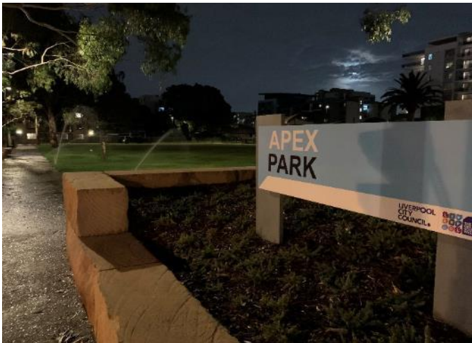
Apex Park Development – Liverpool Council (Automatic Irrigation System)
