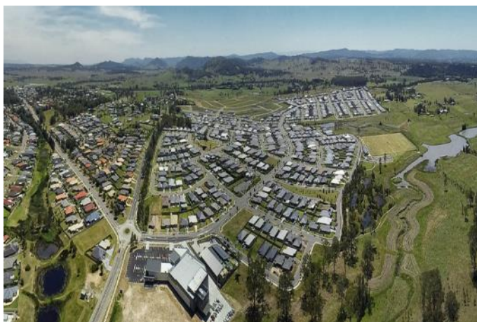
Elara Boulevard, Marsden Park NSW Stockland (Rainwater Basin Recirculation System)
